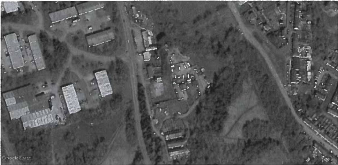
Plate 3: Aerial view of site taken in April 2023 (Source: Google Earth)
