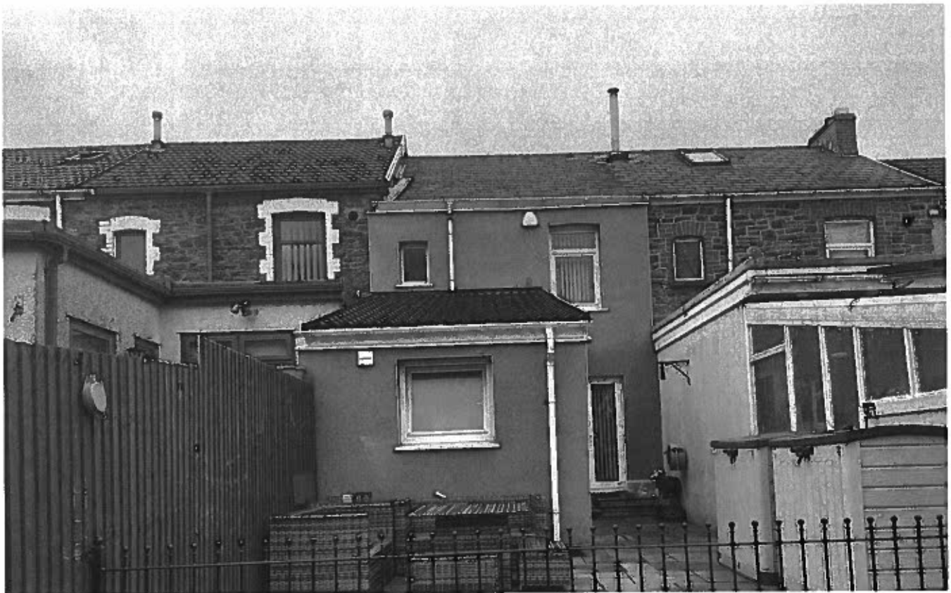
Photo 1 – Rear Elevation of House
