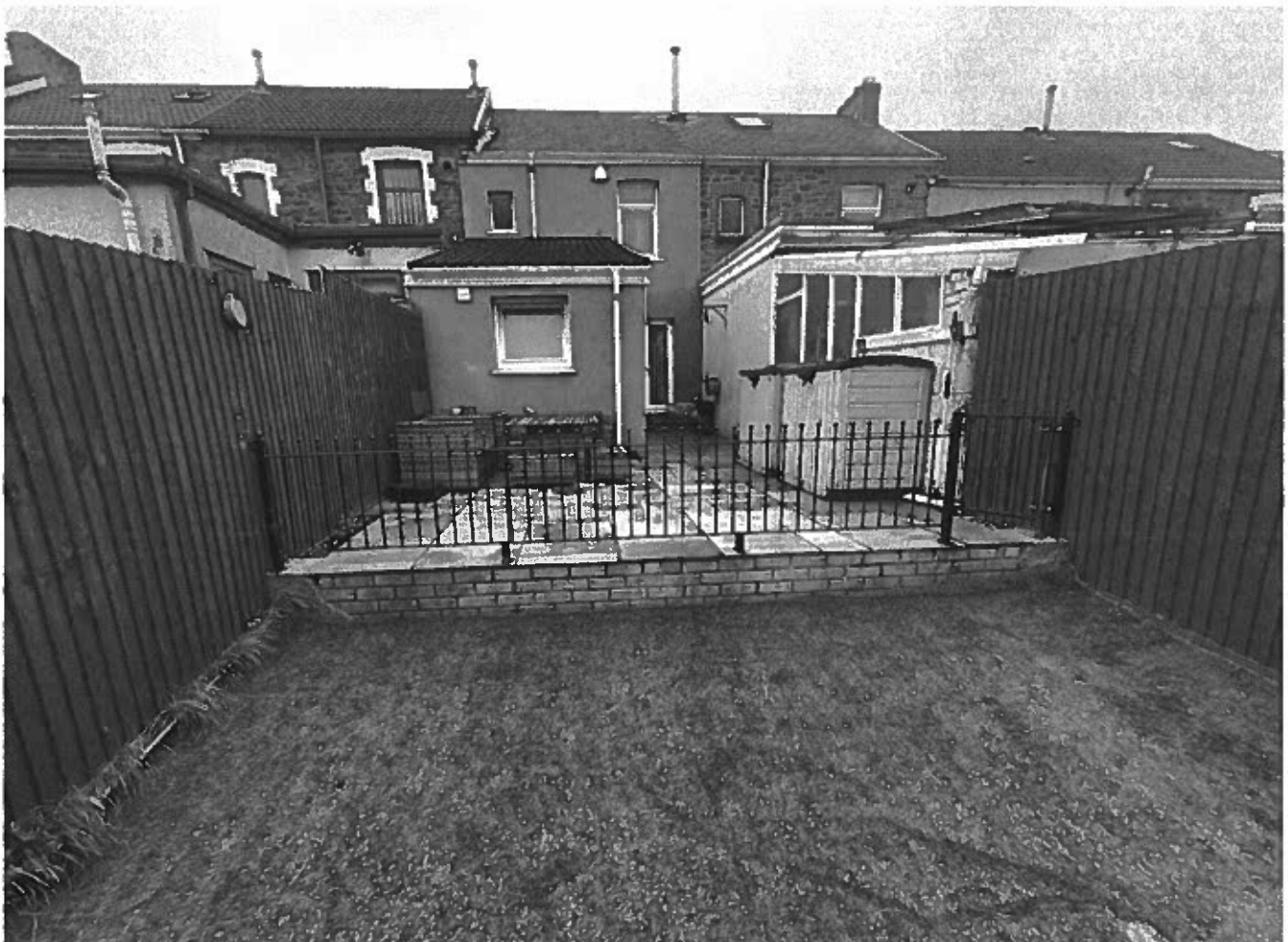
Photo 1 – Rear Elevation of House
