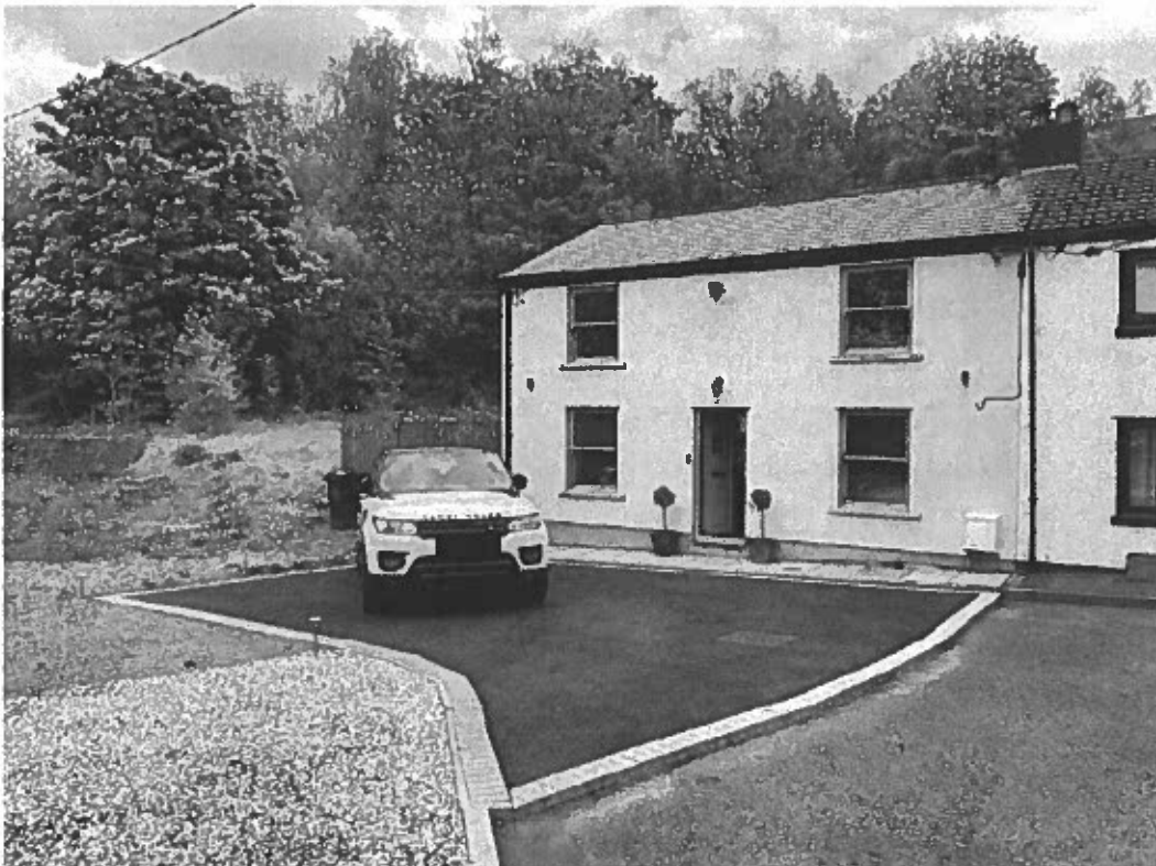
Photo 1 – front of property
