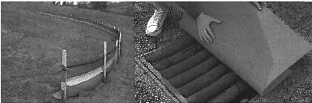
Silt fence (left), road gully filter (right).
